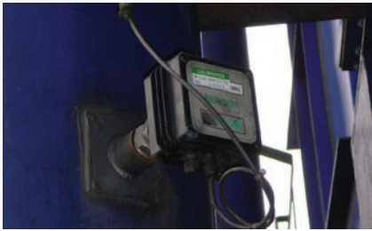
Carbon Black Filter Plant with Electrodynamic Sensors
